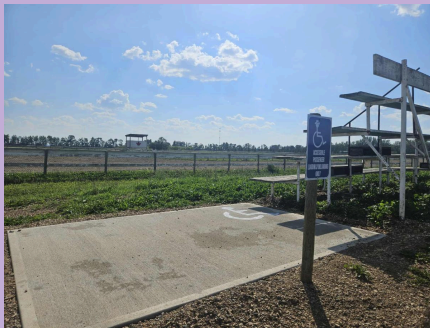
Accessible loading/unloading pad
