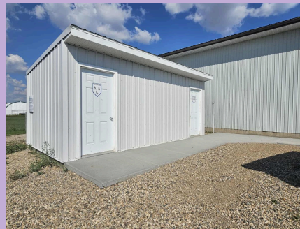
Sidewalk to accessible washrooms
